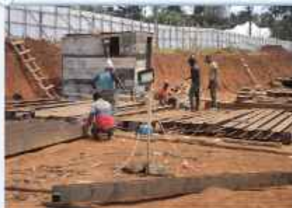
LOT I CUTTING OF I-SECTION COLUMN AND BOTTOM PLATE WELDING FOR TANNERY BUILDING
