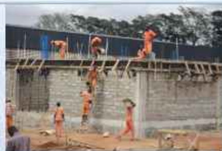
LOT II RING BEAM CASTING OF CANTEEN BUILDING
