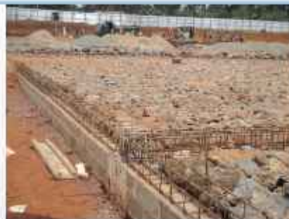
LOT I HARD CORE LAYING AND GROUND BEAM REINFORCEMENT FIXING
